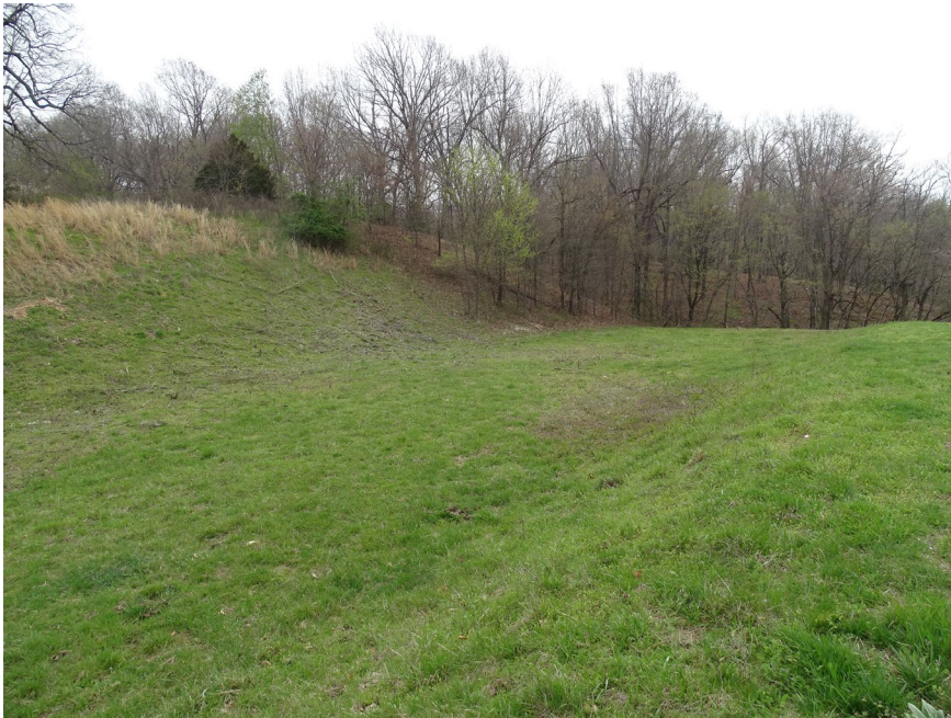
Auxiliary spillway
