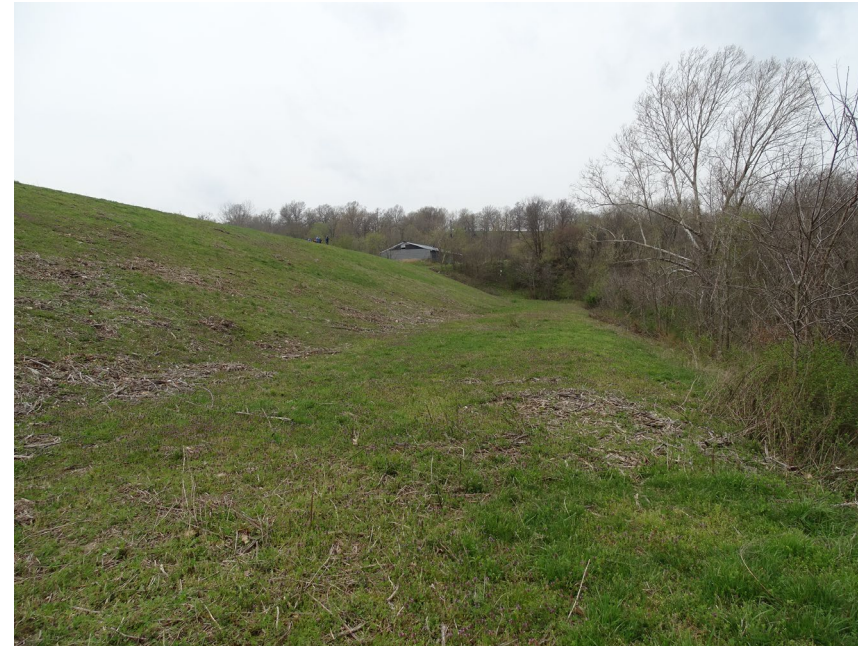
Downstream slope of dam
