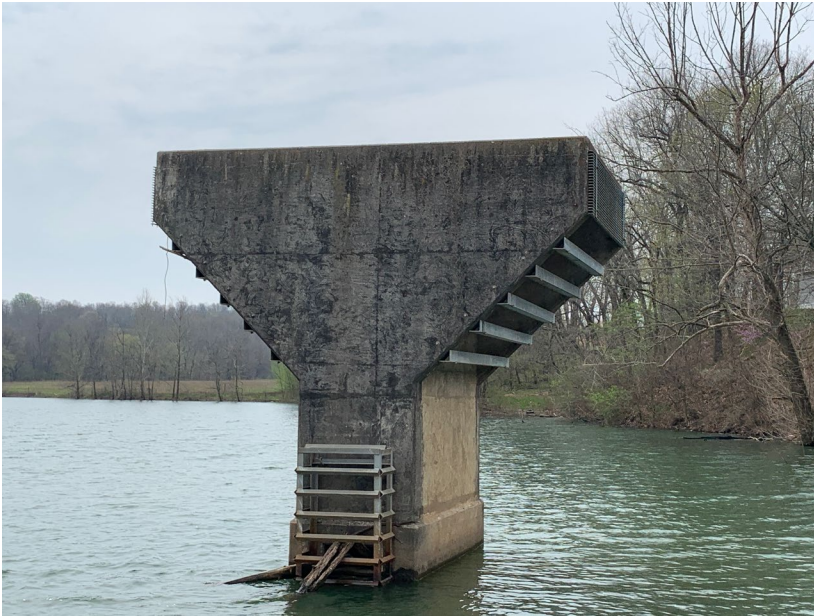
Principal intake structure
