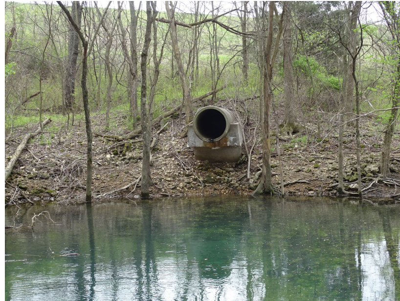
Outfall pipe and plunge pool below dam
