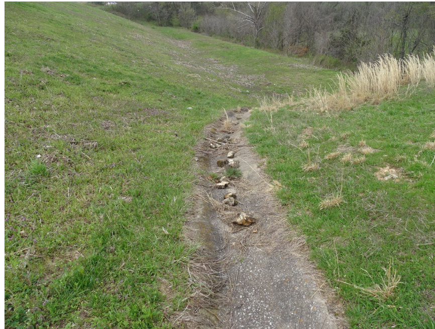
Drainage channel northwest side of dam
