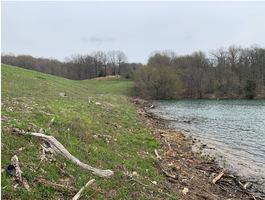
Upstream slope of dam
